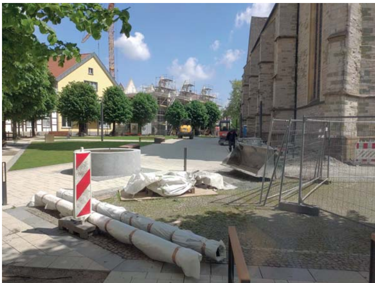
Figure 2. The almost completed St. Stephen's Church Square with upgraded substructure and extended paving (© A. Wunschel, LWL-AfW)
